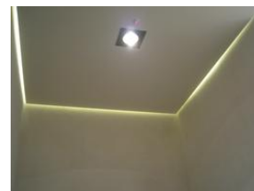
La construction "en action"
