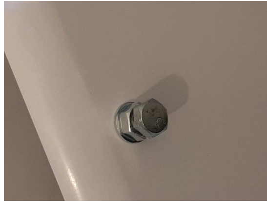
The bolt serves as a convenient handle for the panel door.
