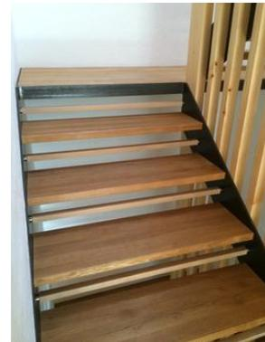
In between each step we now have a wooden bar into which I screwed a GTN-32: Pot magnet with threaded stud  $\varnothing$  32 mm ([www.supermagnete.fr/eng/GTN-32](http://www.supermagnete.fr/eng/GTN-32)) on the left and right. The bar is placed between the steel sides and when in position, the magnets can be unscrewed a little bit and adjusted to sit flush with the steel sides. This way the bars are mounted mechanically and magnetically. Each magnet has an adhesive force of 39 kg!
