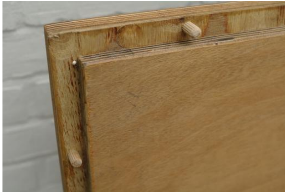
The table top with dowels on the bottom side
